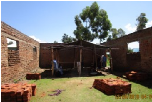
The unfinished building
